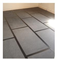
When laid over timber floors airborne insulation up to **43dB** can be expected.
