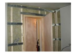
Then install our sound reducing Resilient Bars at 600mm centres across the studwork from floor to ceiling before plaster boarding and as shown in the pic left. To view the technical data on this product please see our Tech Spec page on the website.
