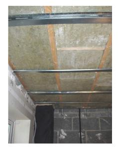
For best results, before the ceiling is replaced, Resilient Bars should be screwed across the joists at 400mm centres as shown above then two layers of high density 12.5mm acoustic plasterboard should be screwed to the bars. An even better result can be obtained if a layer of Acoustic Membrane is sandwiched between the two layers.
