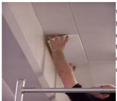
When both surfaces have been properly coated with the adhesive and it has reached the right degree of tackiness, place the panel into position and ensure the tile is properly fixed by pressing with the flat of the hand over the entire surface area of the tile. It is extremely important this is done correctly because failure to do this properly could result in the tile detaching itself in time due to poor adhesion.
