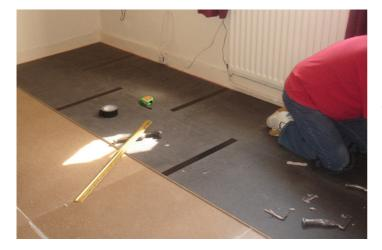
If <u>Soundproofing Mat</u> has been applied first, Quietfloor PLUS edging strips should be fitted against the skirting boards all around the room on top of the Soundproofing Mat then the QuietFloor Plus is installed from the edges of the strips across the remainder of the room as previously described with taped joints. The carpet grippers required for fitting the carpet are then installed on top of the edging strips using longer nails to compensate for the additional thickness.
