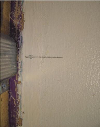
Mark the position of the bars and uprights to help locate them when screwing on the plasterboard. Plasterboard should be screwed to the Resilient Bars with self-drilling screws taking care to avoid hitting the timber stud – **do not screw into the timber stud!**
