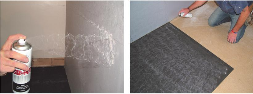
Spray equivalent section of wall for soundproofing mat and also the soundproofing mat with special aerosol adhesive
