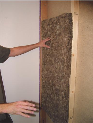
Insert Acoustic Mineral Wool into all of the wall between the timber studs
