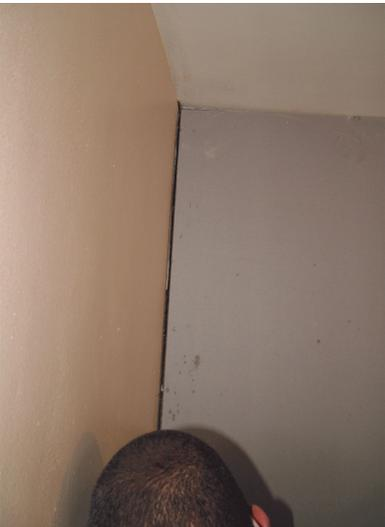
Ensure there is a small gap of up to 3mm around the edges next to floor, wall and ceiling and continue fixing the boards until all of the wall has been covered
