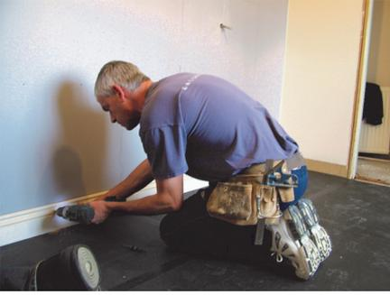
Refit skirting boards by either gluing or screwing. If screwing ensure screws go through to the Resilient Bar and miss the timber framing. Ensure there is a small gap between the floor and corner joints that can be sealed with Acoustic Sealant. Fit surface mounted electrical fittings and the sound insulated wall is finished except for decorating
