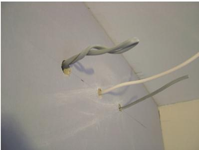
Holes allowing for electrical wiring should be sealed with Acoustic Sealant
