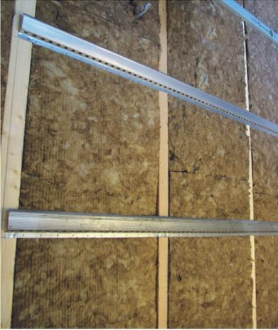
Install Resilient Bars at 600mm centres from floor to ceiling
