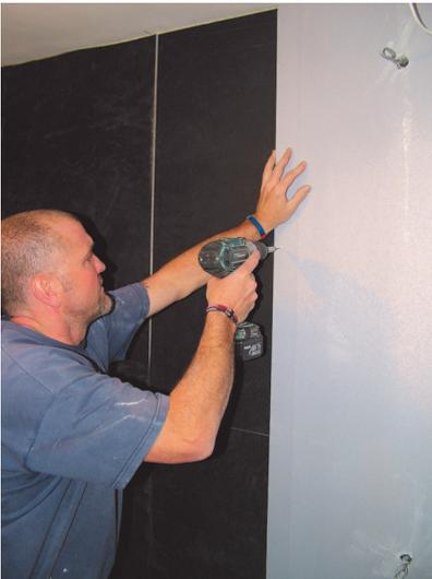
Fix second layer of acoustic plasterboard maintaining the small gap between the floor, walls and ceiling using spacers as necessary. Use the marks previously made to help position the screws and ensure they do not come into contact with the timber frame. Tape and finish off the joints
