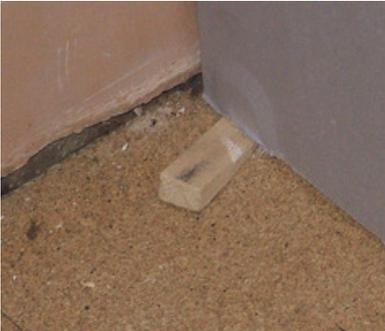
Screw on first layer of acoustic plasterboard with a small gap around the edges of the floor, walls and ceiling using spacers at floor level as shown
