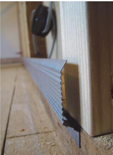
Fix Resilient Bars across the timber stud with the fixing flange on the bottom edge as shown. The bottom and top rails should have the ribbed section fitted clear of the top and bottom plates
