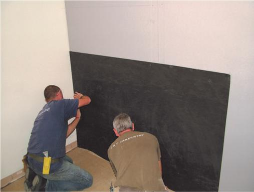
Immediately stick the soundproofing mat onto the glued section of wall ensuring there are no air bubbles and continue until the entire wall has been covered with joints butted to one another. Do not leave overnight but fix the second layer of plasterboard as soon as the mats have been glued on.
